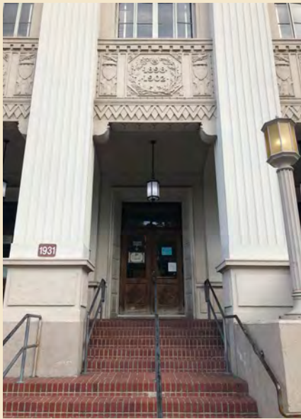
Figure 6.4 Spandrel panel with the dates of the Spanish American War.
