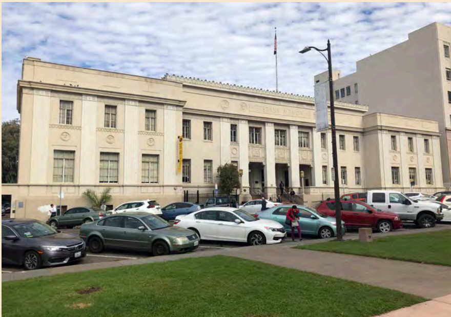
Figure 6.1 Front (south) façade with three-part composition.
