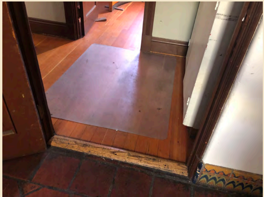
Figure 7.23 A wood floor installed over the original floor in the first floor Vestibule creates an inaccessible door threshold.
