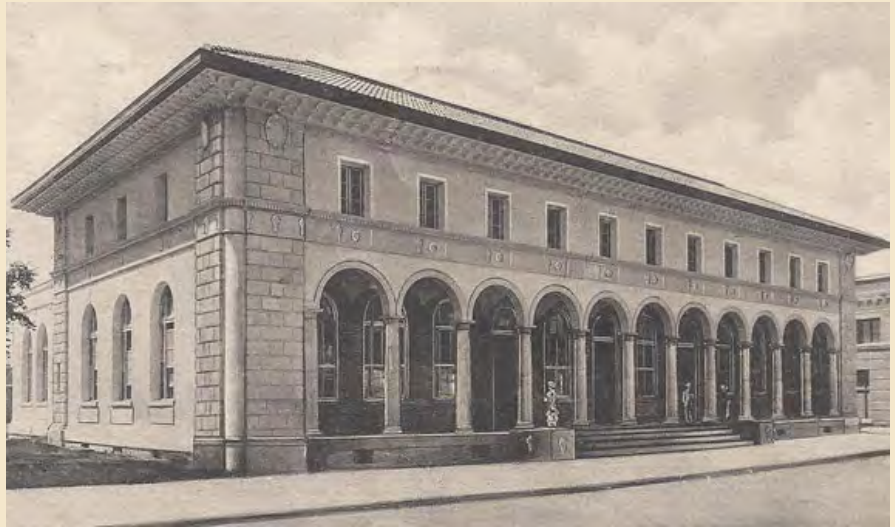
Figure 4.3 Berkeley United States Post Office, completed 1914, by architect Oscar Wenderoth; modeled after Brunelleschi's Foundling Hospital in Florence. Source: Historic Postcard.
