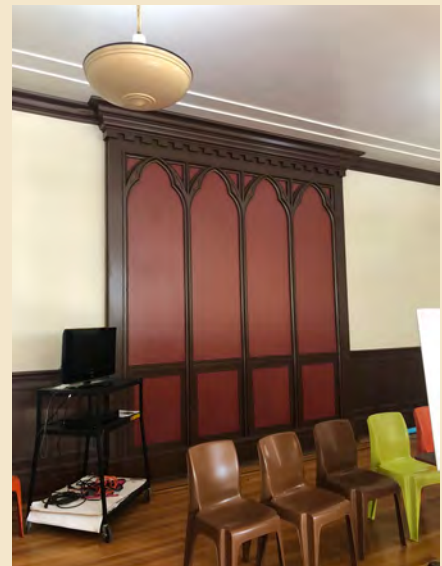
Figure 7.26 In Lodge Room #1, the decorative wood paneling may have originally been painted with decorative stenciling.
