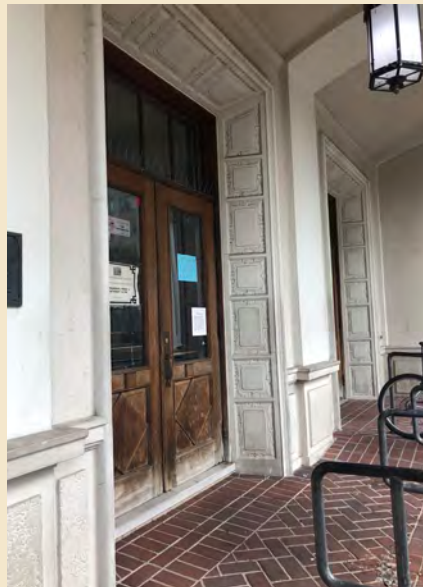
Figure 6.3 The entrance vestibule has three pairs of wood entrance doors surrounded by doorjambs with panels and stylized arabesques.
