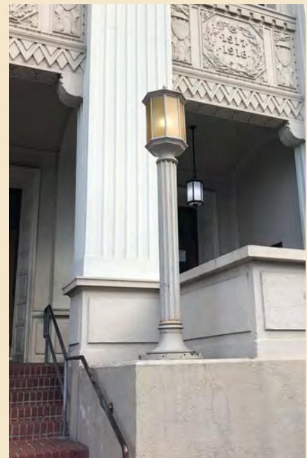
Figure 6.10 Fluted metal light posts topped by amber-glass lanterns flank the main entrance stairway.
