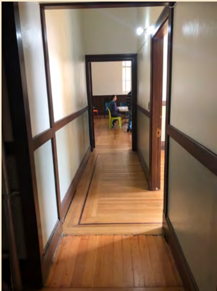
Figure 7.24 The Women's Rest Room has been divided to create a new entry hall to Lodge Room #1.
