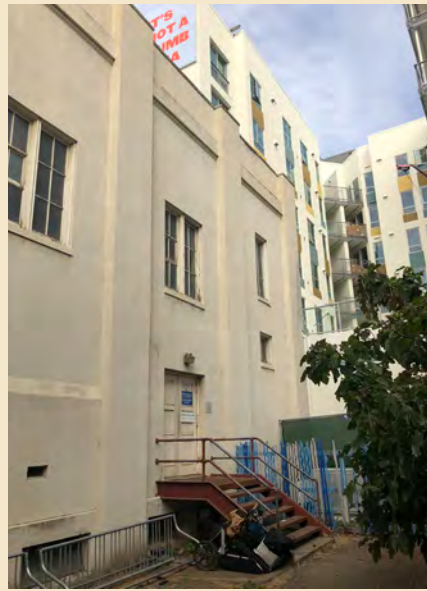
Figure 6.8 The rear elevations are utilitarian in appearance.
