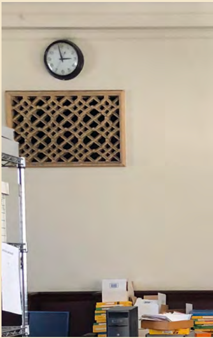
Figure 6.24 Vent grilles at second floor.
