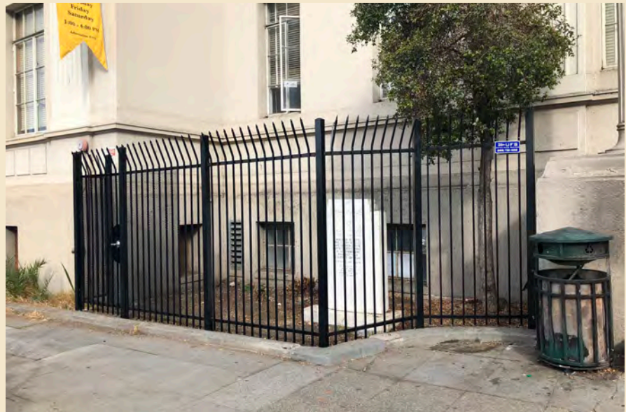
Figure 7.1 A recently installed metal fence at the primary façade is incompatible with the building.
