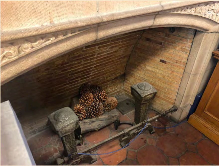
Figure 6.22 Original fireplace in the former Men's Club Room (now the Berkeley Historical Society).
