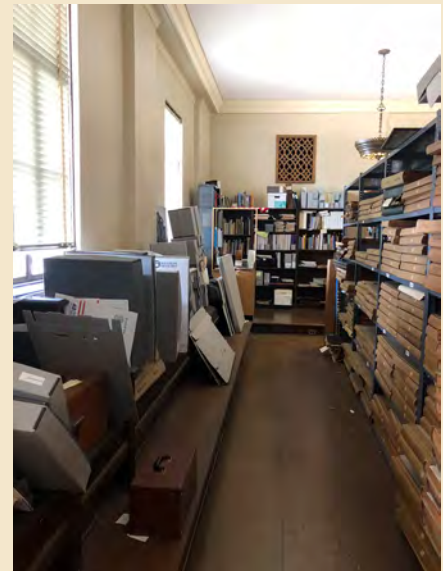
Figure 7.37 The original built-in platform and benches in Lodge Room #3 are intact. The linoleum flooring seen here may not be original as the building specifications called for maple flooring in this room.
