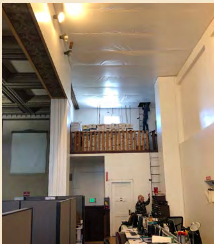
Figure 7.18 The stage within the auditorium is currently used as office space.
