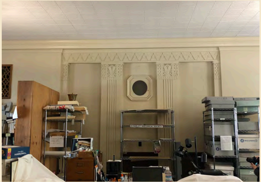
Figure 7.35 The decorative plaster wall paneling at Lodge Room #3 would likely have been different colors originally.
