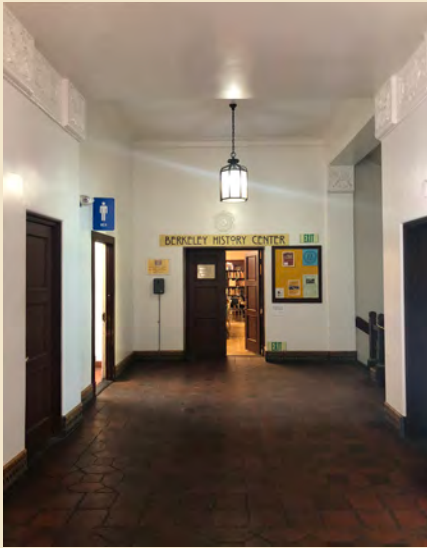
Figure 7.10 The building lobby features the original Gladding McBean terra cotta tile floors, Solon and Shemmel polychrome wall base tile, among other finishes. The walls and ceilings may have originally been painted with decorative stenciling.
