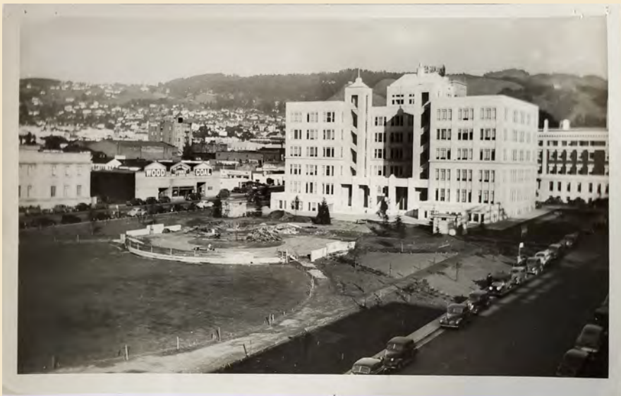
Figure 4.9 Federal Land Bank Building with the Civic Center Park fountain under construction, 1941-42. Source: Berkeley Architectural Heritage Association.
