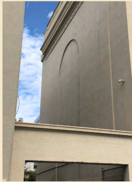
Figure 6.12 Two-story, semicircular blind arch.
